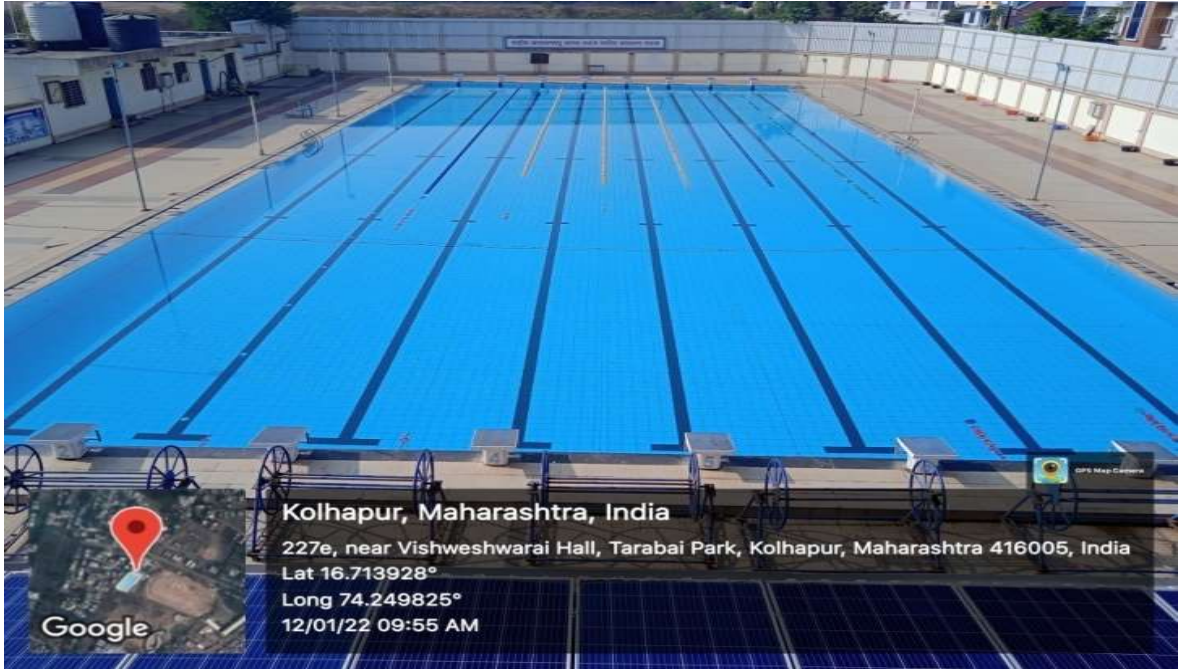
Swimming Pool facility
